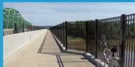
Shared use path on the I-64 Boone Bridge.
