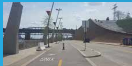
Leonor K Sullivan Blvd raised cycle track
