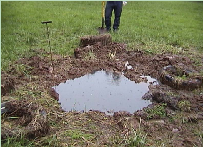
Overflowing septic tank.
