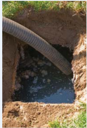
Septic tank pump-out.
