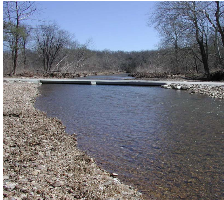
Fish-friendly low water crossing
