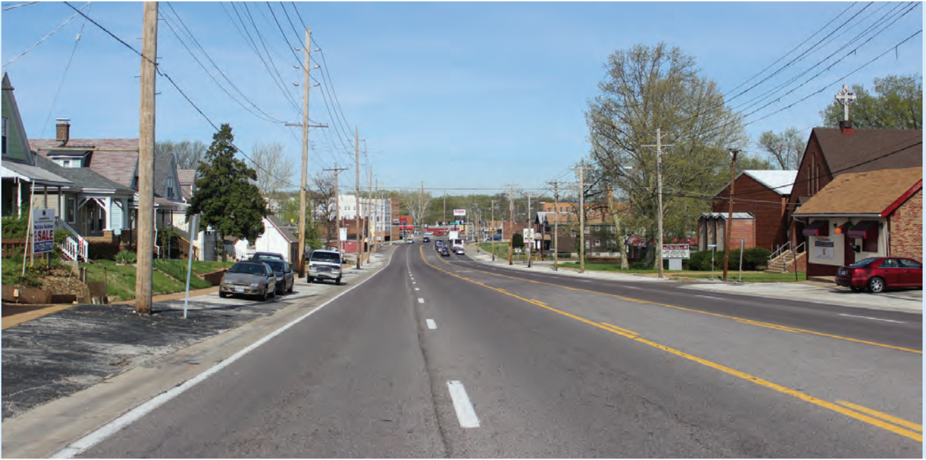
PHOTOGRAPH OF EXISTING CONDITIONS ON PAGE AVENUE
