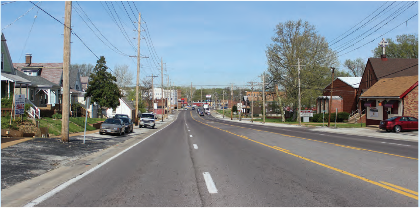
PHOTOGRAPH OF EXISTING CONDITIONS ON PAGE AVENUE
