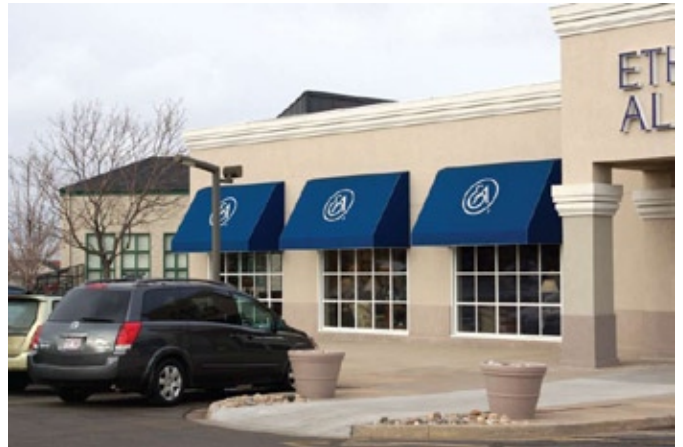
Example of an Awning Sign
