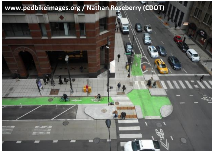
Figure 16: Protected intersection utilizing colored pavement and curb bump-outs to increase visibility and reduce crossing distance for people walking and bicycling
