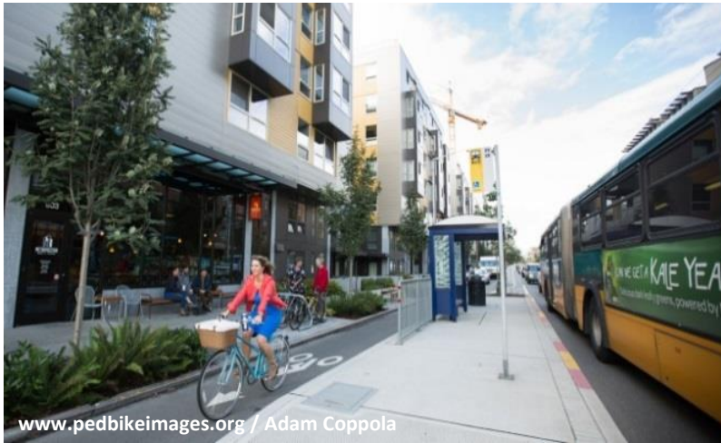
Figure 18: Public transit is separated from bicycle traffic with a raised bus stop, allowing bicyclists to continue through the bike lane without interruption as buses stop for passengers
