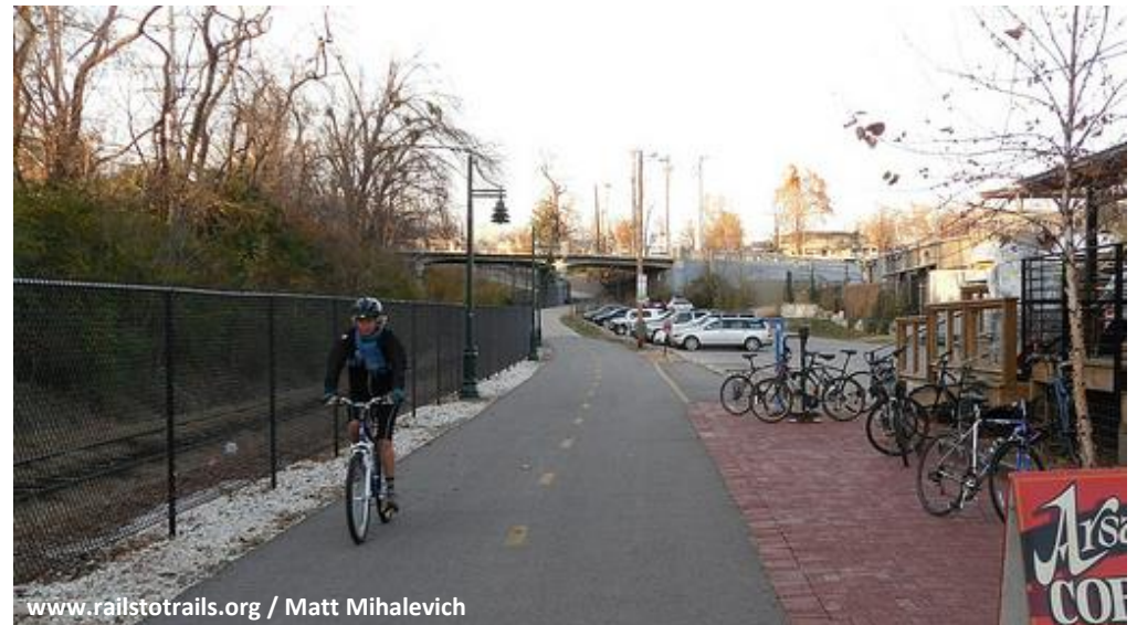
Figure 19: Fencing is used to separate the railroad from the bicycle facility
