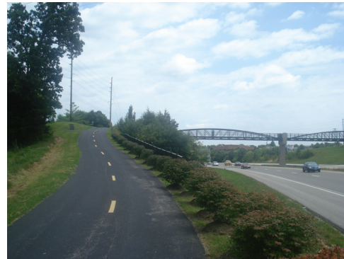
Existing Pedestrian / Bicycle Trail Along Route 100 and Pedestrian Bridge, Wildwood
